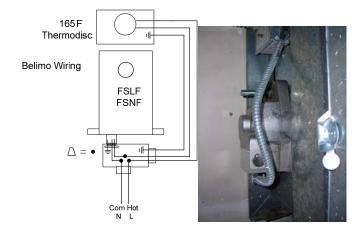
For short shaft mounting, the ZG-LMSA-1/2-5 can be used. Alternately, the clamp can be installed between the actuator and sheet metal.
