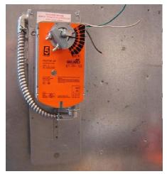
On small dampers the actuator may be hung out in the air. The duct must be able to fall away, so actuator cannot be attached to the duct.
