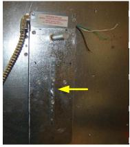
On small dampers the actuator may be hung out in the air. The duct must be able to fall away, so actuator cannot be attached to the duct.
